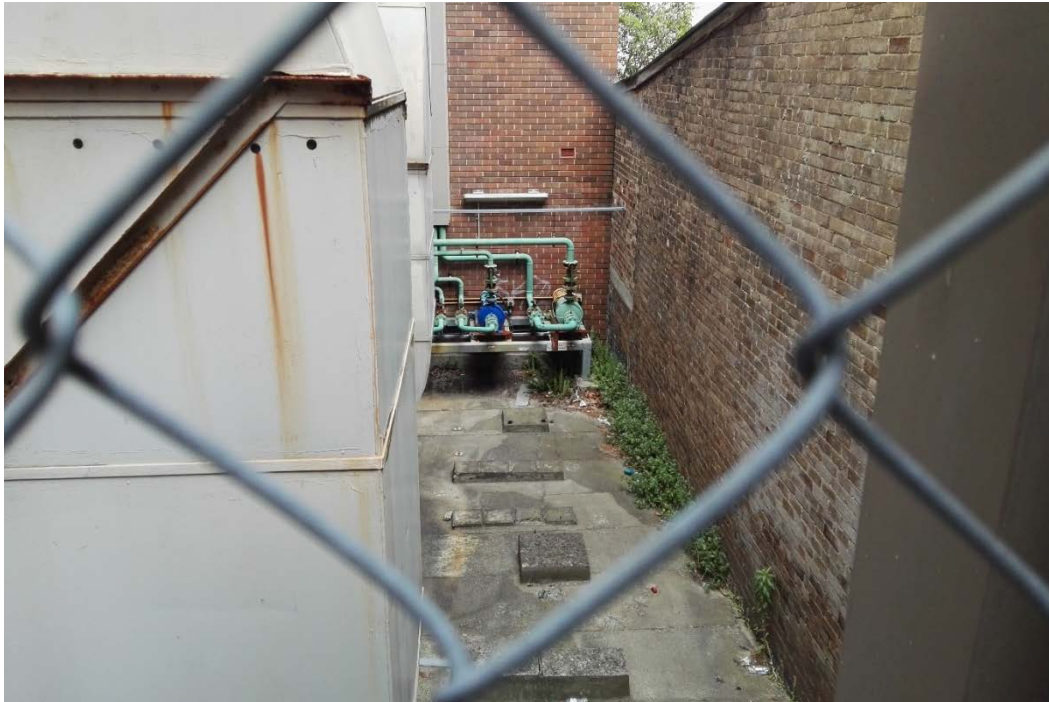
Photograph 6: Secure concrete compound containing pipework. Signs indicated that the pipework was decommissioned.
